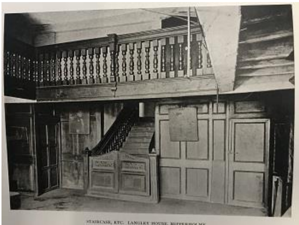
STAIRCASE, ETC. LANGLEY HOUSE, HIPPERHOLME
